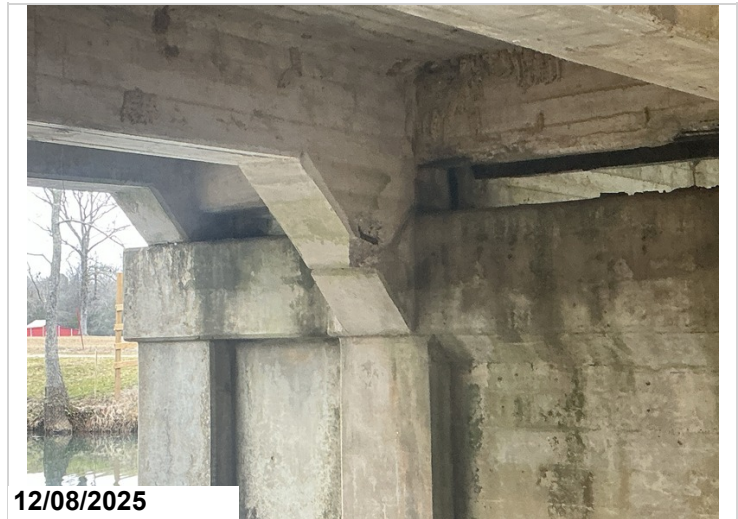
Span 1, girder 2, at bent 2: small spall with exposed rebar. CS3-1'
