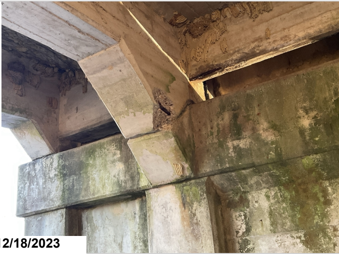
Span 1 bent 2 girder 2 right side spall with exposed rebar at girder haunch. 8" x 8" x 1" deep.
