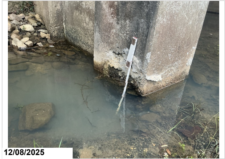
Bent 4, column 1: bottom of column with a spall. CS3-1
