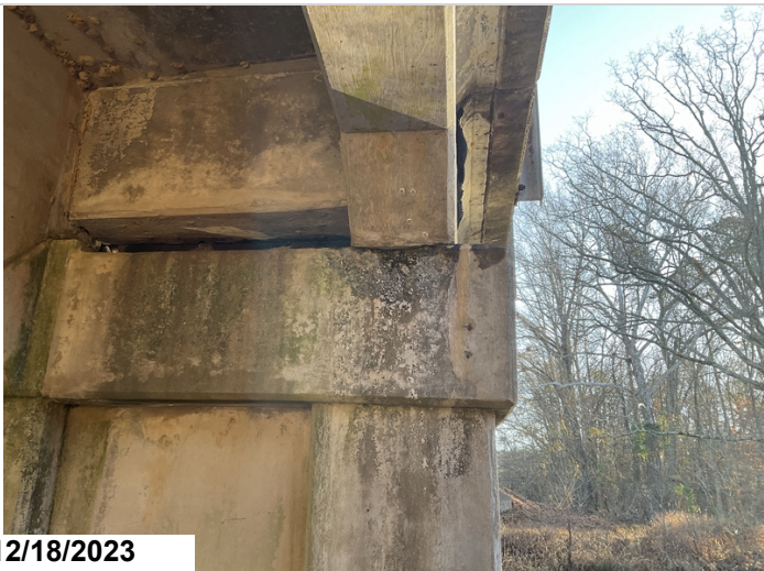
Bent 2 pier wall back small spalls with exposed rebar & delamination under girder 5. 1' x 8"x 2" deep.
