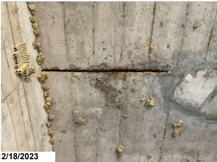
Span 4 between girders 3 & 4 spall with exposed rebar in the soffit. 3' x 1" x 1/2" deep.
